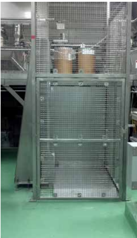
FRONT LOWER ENTRANCE DOOR CLOSED
