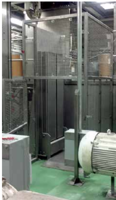
FRONT LOWER ENTRANCE DOOR OPENED
