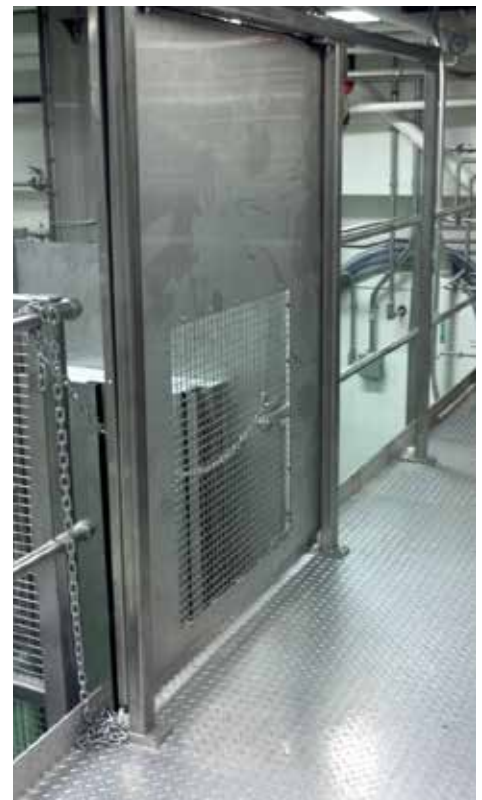
REAR UPPER ENTRANCE DOOR INSTALLED & CLOSED
